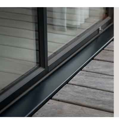
Outer frame sill channels have drain holes that can become clogged with paint, grime or insects. Clean them out and keep them open to ensure that the windows maintain their designed weather performance.
