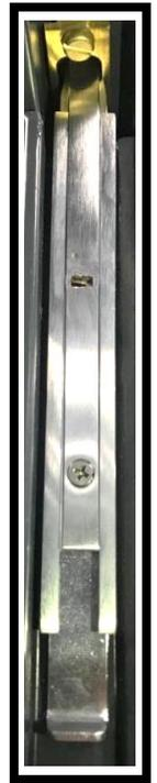
For double leaf doors, there will be a handle and locking system on the master leaf. On the slave leaf, there will be a concealed bolt which will enable the door to remain shut when unused and also have the ability to open and to maximise space. These are key operated. Please see image to the right.
